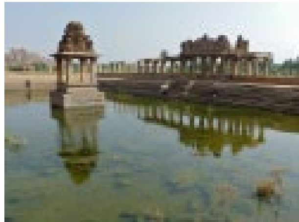
Tank at Hampi, ASI monument number N-KA-B49. Loss of maintenance in original stone aqueducts and intake channels has left historic basins dry or improperly drained, causing uneven thermal expansion and contraction in the stone tiers. Unregulated tourist movement, accidental abrasion, and climbing on delicate historic masonry has accelerated surface wear throughout. Photo by Jonathan Freundlich, 13 November 2011, 10:36:53 Creative Commons Attribution-Share Alike 3.0 Unported license.
