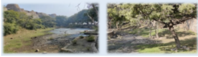
INDIA TUGHLAKABAD FORT, DELHI. THE MUNICIPAL AGENCY ENCROACHED THE SITE BY DRAINING SEWAGE WATER INTO THE PROTECTED AREA OF THE MONUMENT. 2022 PERFORMANCE AUDIT PHOTO.
